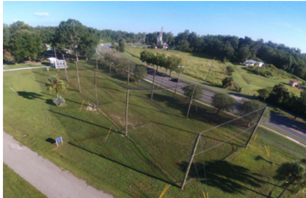
Figure 2-1. Aerial view of the Autonomy Park netted enclosure.
